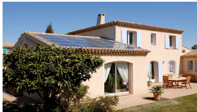
Figure 14 – Example of an excellent installation with PV modules integrated in the rooftop
